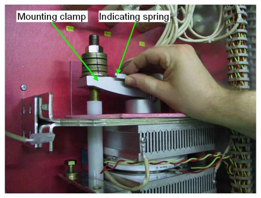
5. Loosen the mounting clamp at the top of the thyristor stack.
