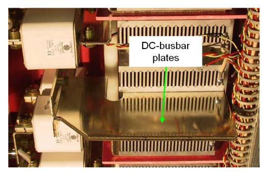
7. Attach the disassembly tool at the faulty thyristor and prize open the upper and lower heat sinks.
